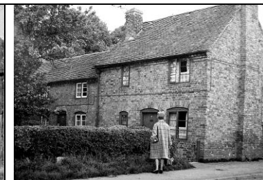
Far left: The Roberts family outside their cottage, demolished in 1950. Left: Nos 8 & 10 Chapel Street in 1968, moved from Evesham in the 1850s.
