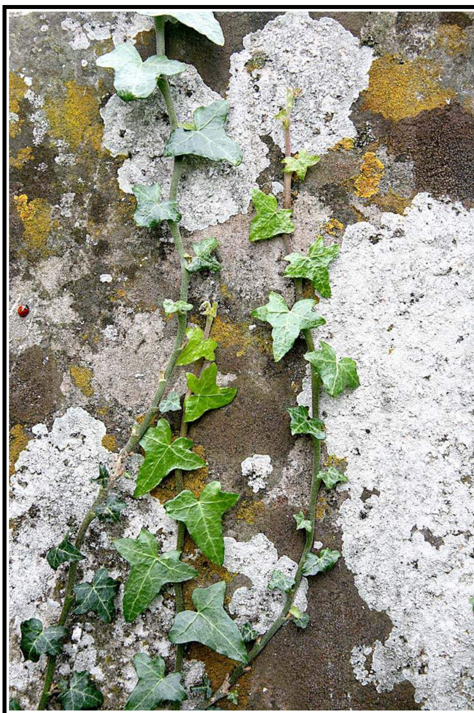
Ivy on a headstone. Probably the most invasive and destructive plant to be found in the churchyard and should be removed before it has chance to invade the cracks in the stone and cause permanent damage.
